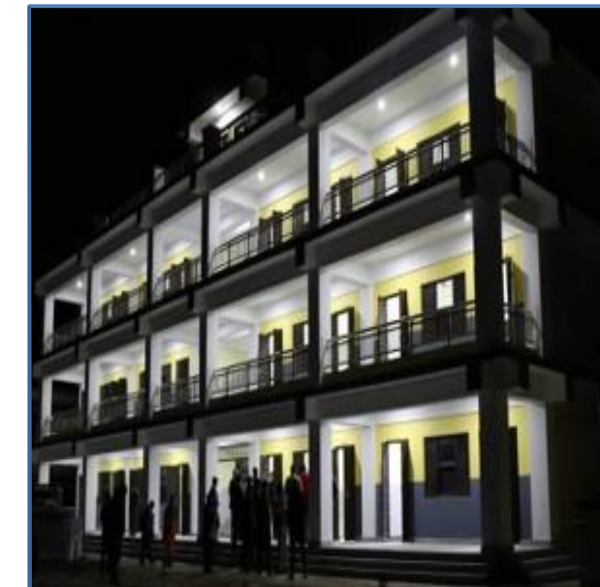
Reconstructed School Building Post Earthquake
